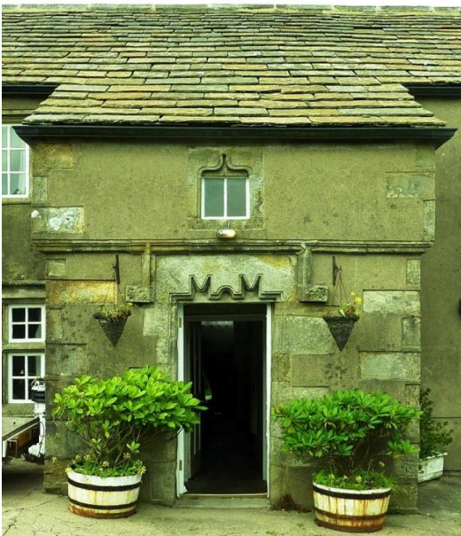
Illustration 3. Higher Stony Bank jettied porch. Note monopitch roof and other decoration, including ogee-headed porch window. Photo K.I.
